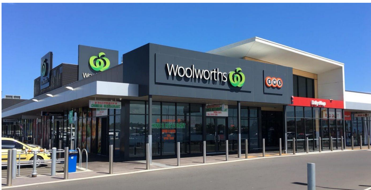
Exterior of Dalyellup Shopping Centre
